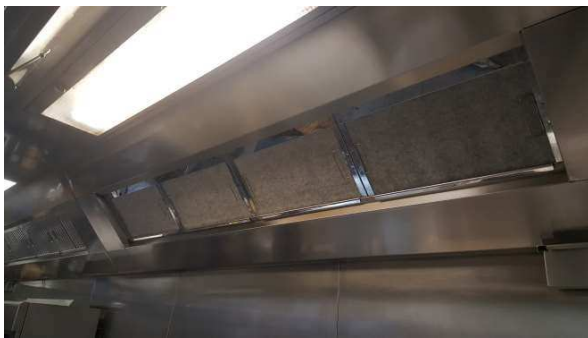
New Filters Installed.
